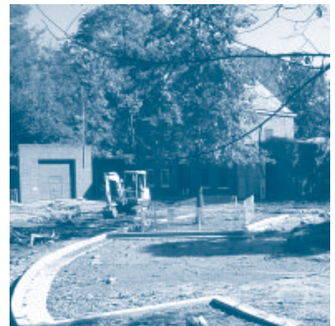
Permeable paving installation at Back Creek Nature Park, Fall 2008
